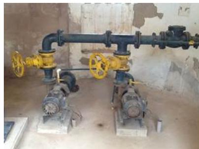
**Figura 0.42 – Bomba Recalque
